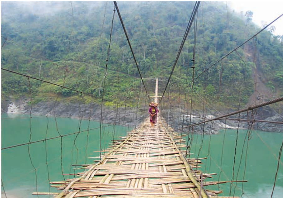
The pace of life in rural Arunachal Pradesh, where local people use such bamboo suspension bridges to connect from their remote villages to the main road. (Photo by Mirza Zulfiqur Rahman.)
